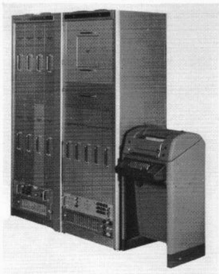
Figure 9. Display Control Cabinet and Printer
